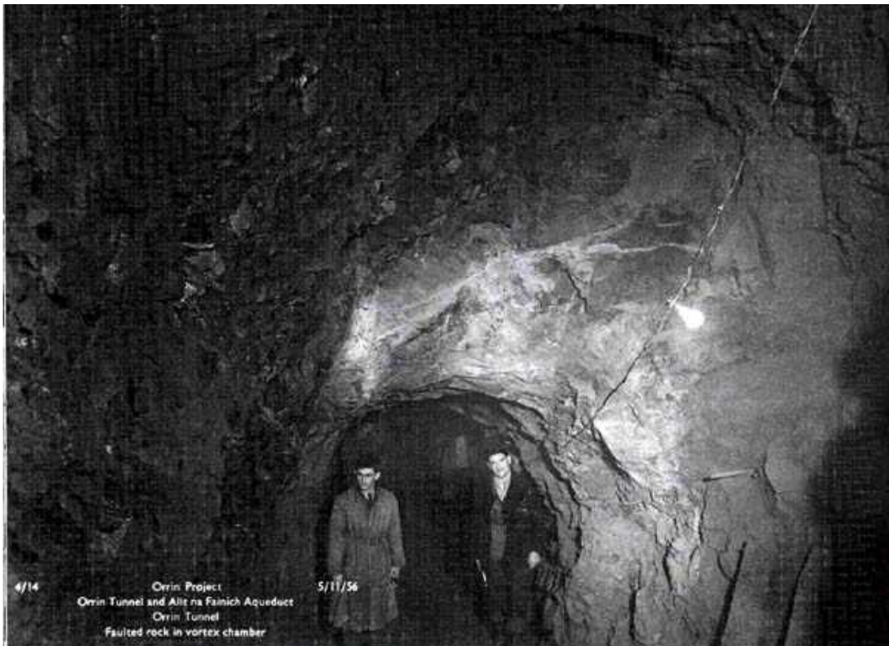
A rock fault in the Orrin tunnel (NOSHEB)
