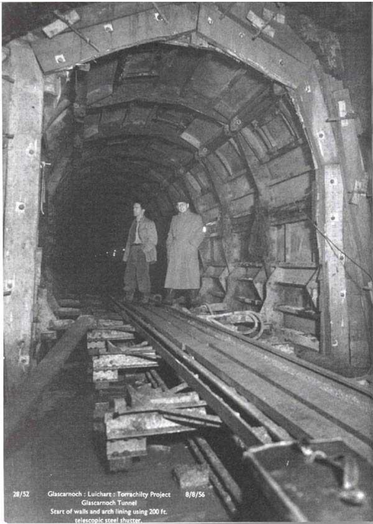
Glascarnoch tunnel. Start of walls and arch lining using a 200 foot telescope steel shutter, August 1956 (NOSHEB)
