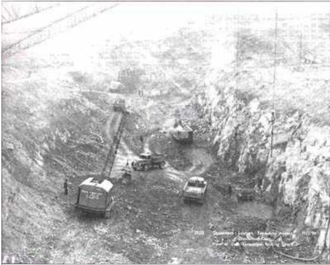
Excavating the foundations for the Glascarnoch dam, March 1954 (NOSHEB)
