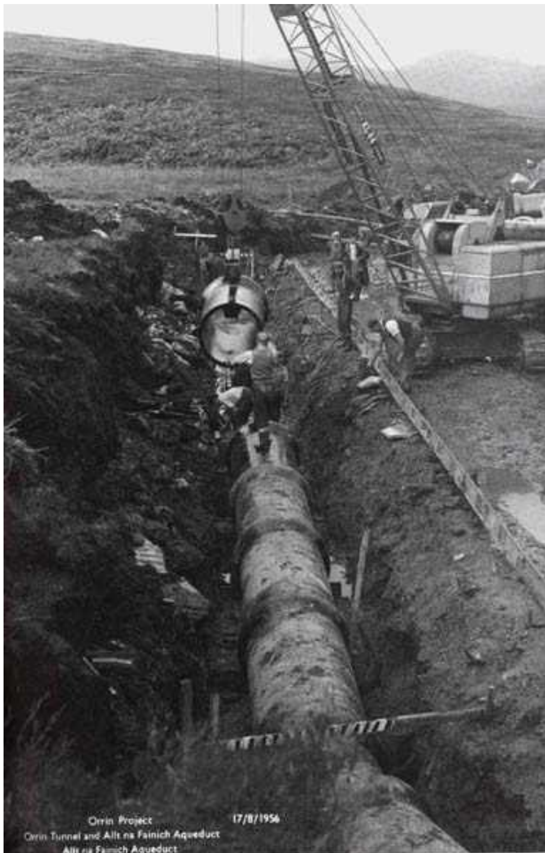
Laying the Allt a Fainich aqueduct on the Orrin scheme, August 1956 (NOSHEB)
