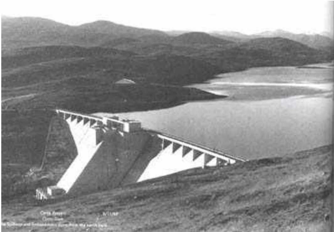
The completed Orrin dam, November 1960. The fish pass is in the sloping concrete structure in the centre (NOSHEB).
