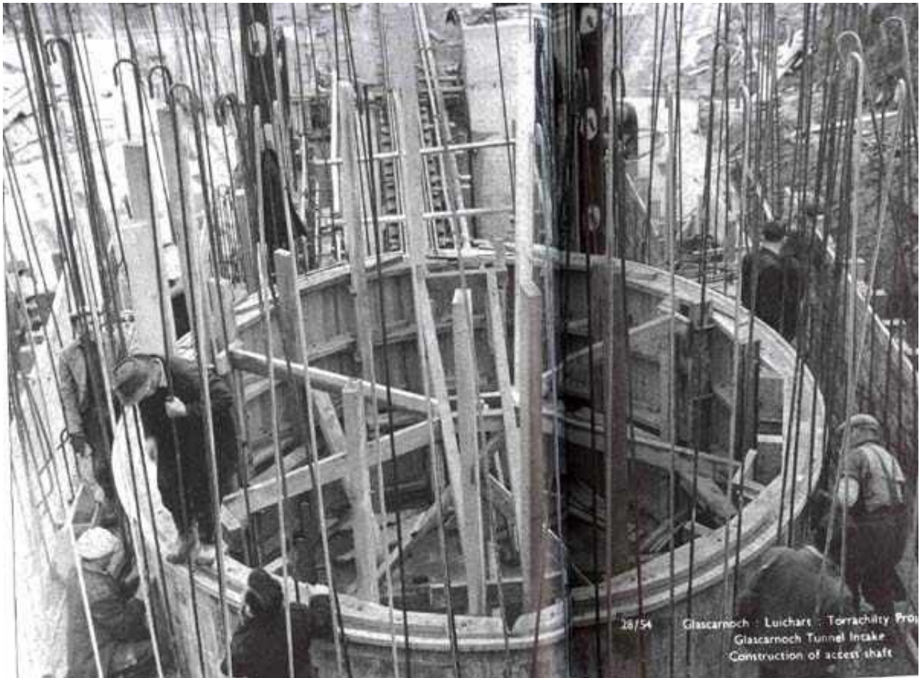
Constructing the access shaft to the Glascarnoch tunnel intake, September 1956 (NOSHEB)
