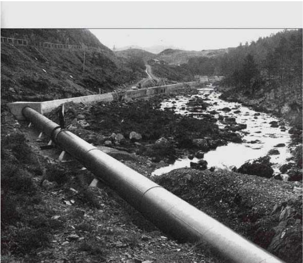
The pipeline following the Kerry river, Gairloch, from the reservoir to the power station, May 1951 (NOSHEB)
