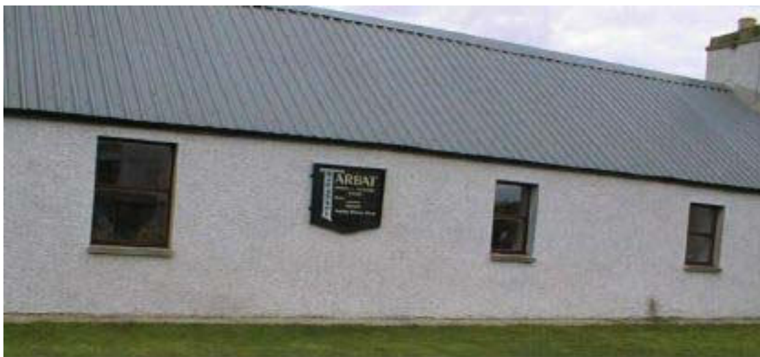
Inver Meeting House in 1998 with windows and a waterproof roof.
