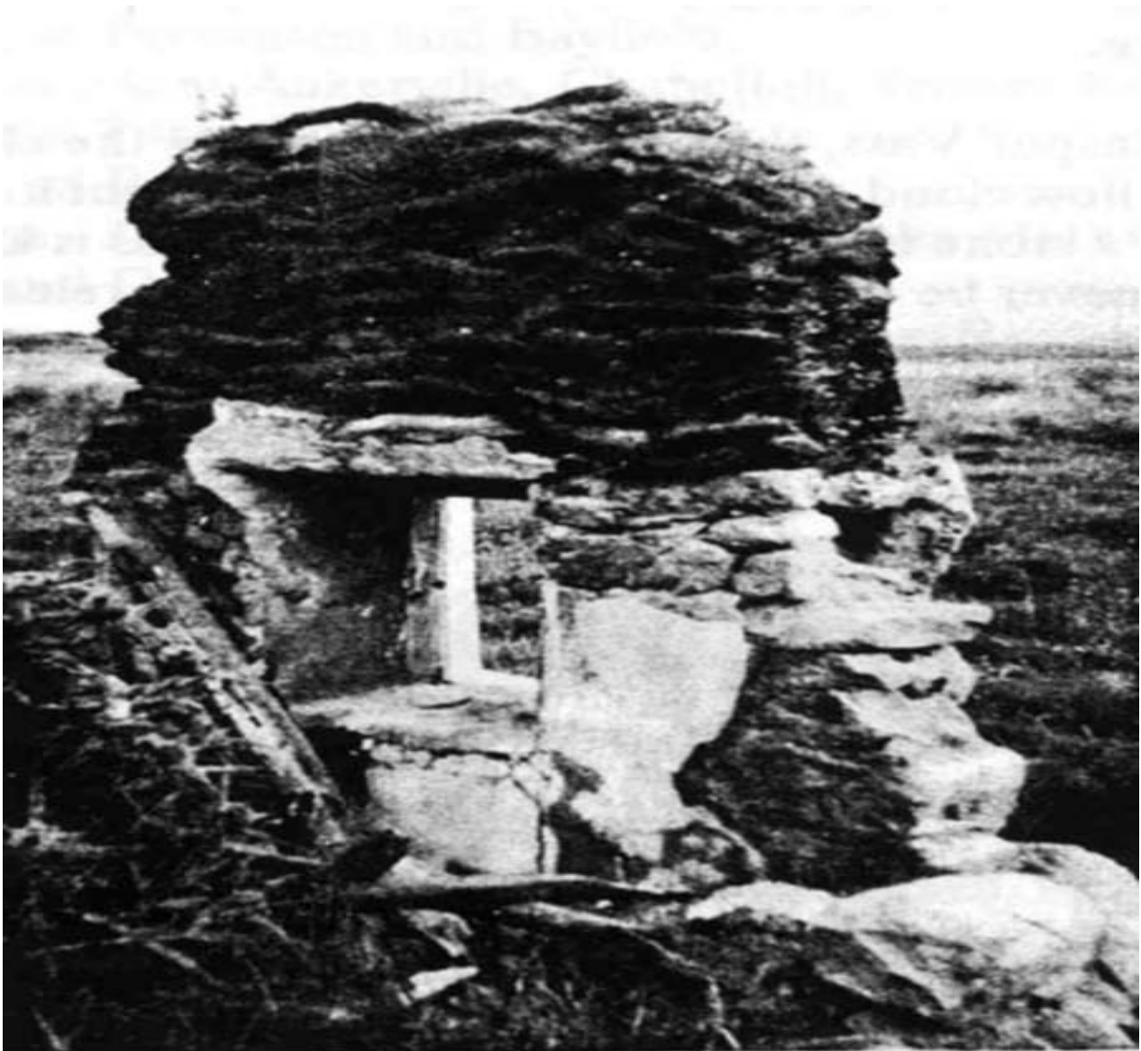
House at Balnapaling showing use of turf in walls.
