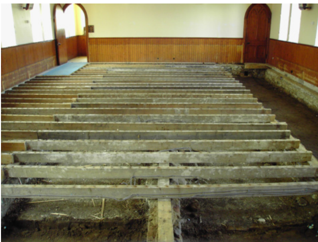
Asbestos-covered pipes removed. The joists are
