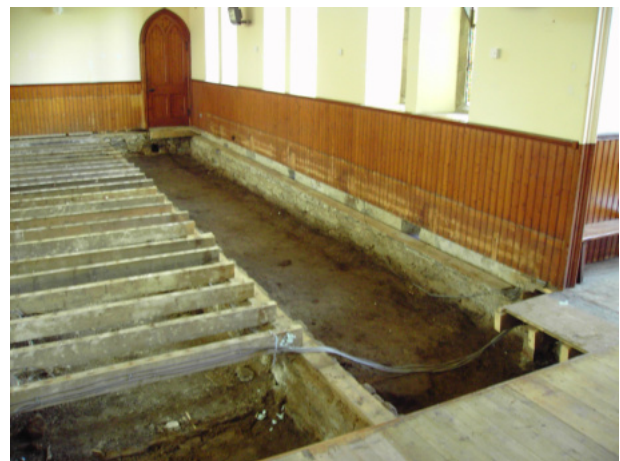
Area awaiting new joists.
