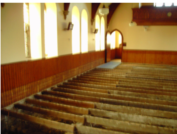
Very few joists requiring attention on this side.
